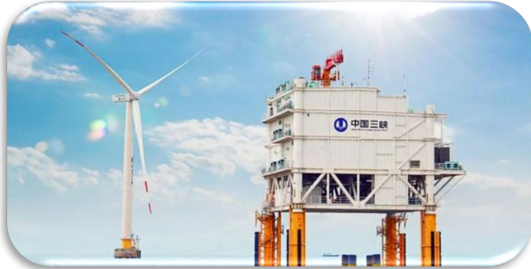
Converter Substation Floatover
